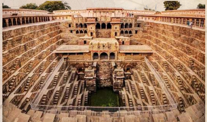
Chand Baori Stepwell, Rajasthan The stepwell was built 1000 years ago highlighting 3500 steps, 13 stories, and 30 meters underground.
