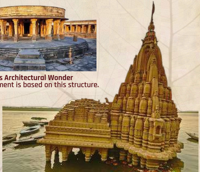
Ratneshwar Mahadev Mandir Varanasi, Kashi Stands 74 meters tall, tilting at a 9-degree angle, it's submerged in the Ganga river for 6 months yearly. In comparison, the 'Leaning Tower of Pisa' tilts 4 degrees and is 54 meters high.
