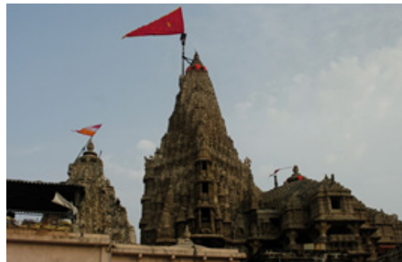
Figure 30: Temple Steeple Dwarka
